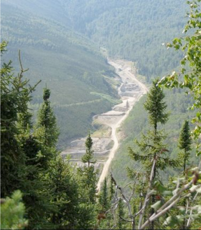
Narrow valleys utilise mined out areas downstream as settling ponds
